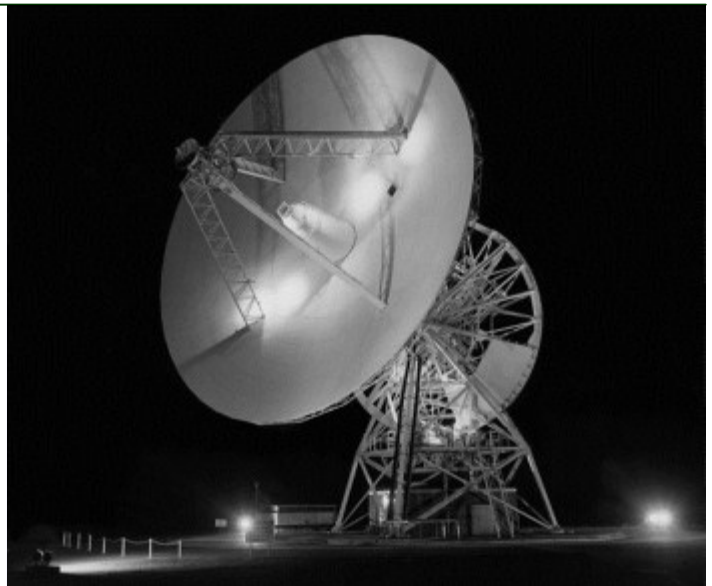
The Honeysuckle antenna by night. Photo by Hamish Lindsay.
